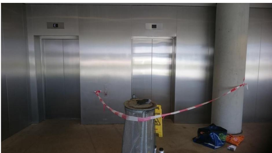
Hamburg Airport Parkingdeck P1 ground zero. Left door is untreated, right door is treated with nC Protect 4600 PT Finish. Picture shows situation 1 week after treatment. Application was done by cloth and sponge. (picture R. van Hoorn)
